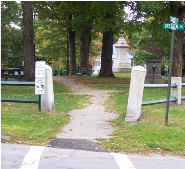
Existing entrance condition
