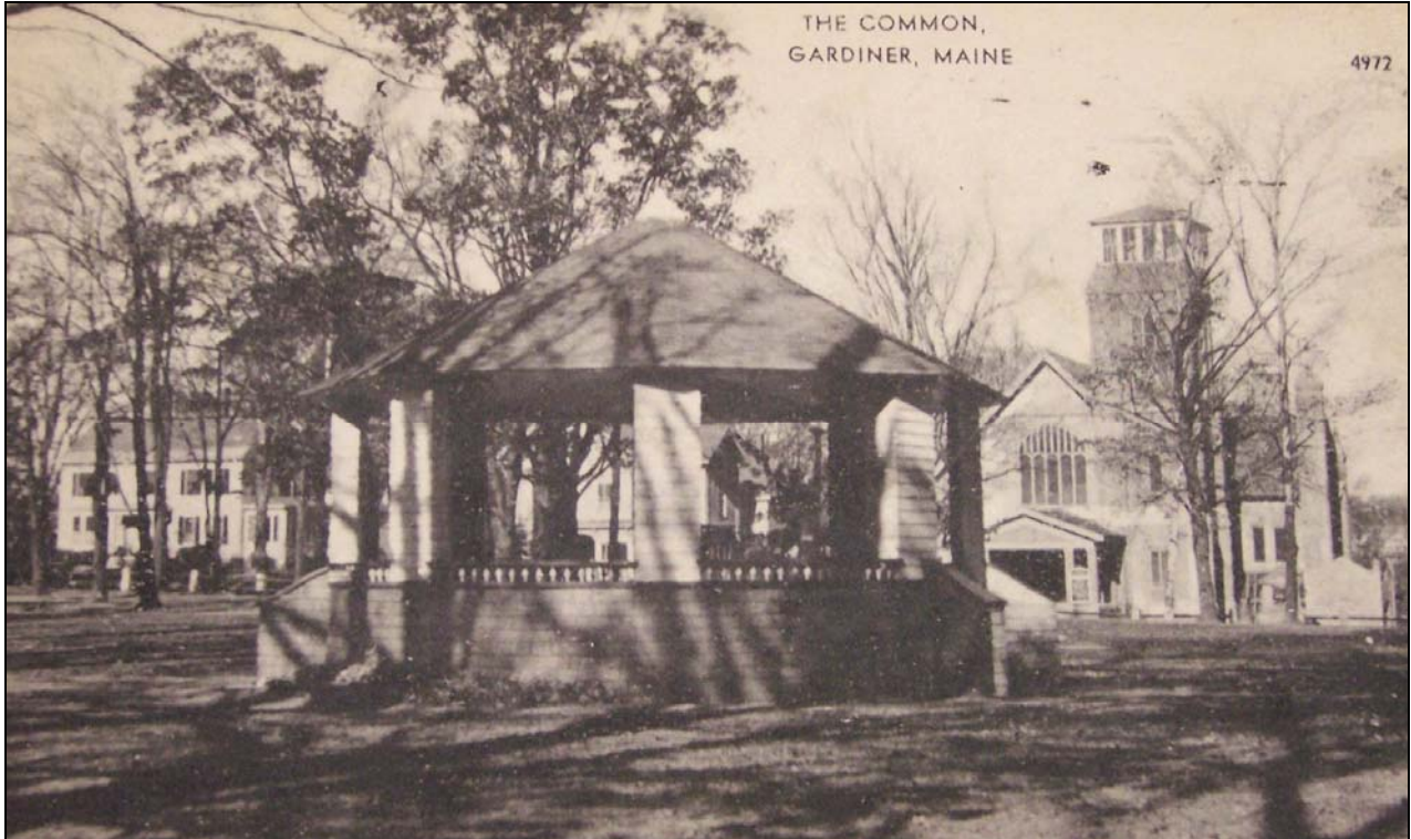
Historic shingle-style gazebo.
