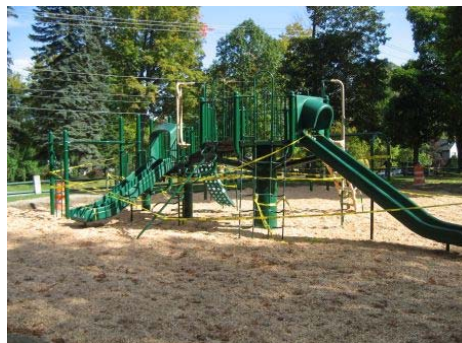
New Gardiner Playground Under Construction-Oct, 2009
