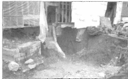
Photo 3 - Excavated hole and exposed foundation
