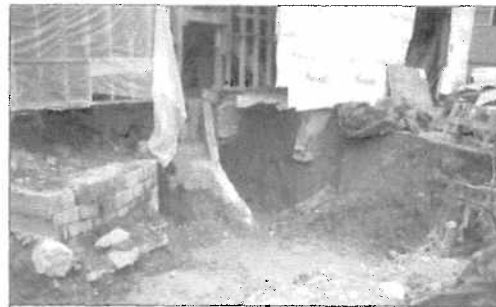
Photo 3 - Excavated hole and exposed foundation
