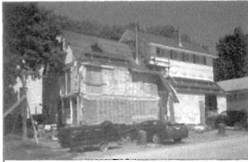
Photo 1 - View of house from Clinton Street
