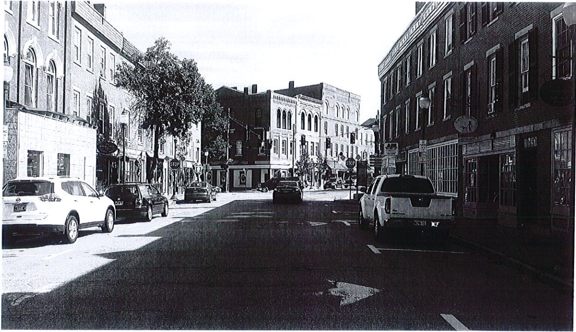
Water Street eastbound
