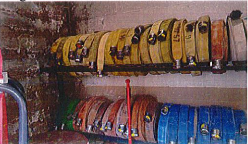
Hose Tower (Fire Dept)
