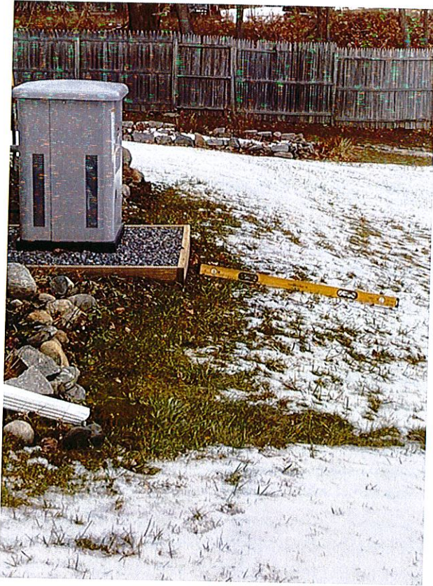
Opposite end of house showing grade
