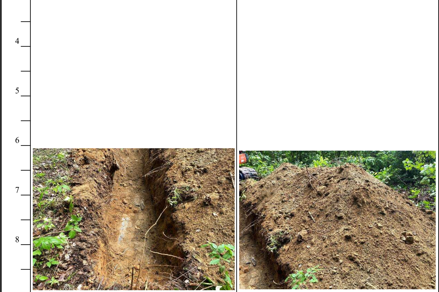
Photographs showing the test pit excavation and soil profile.
