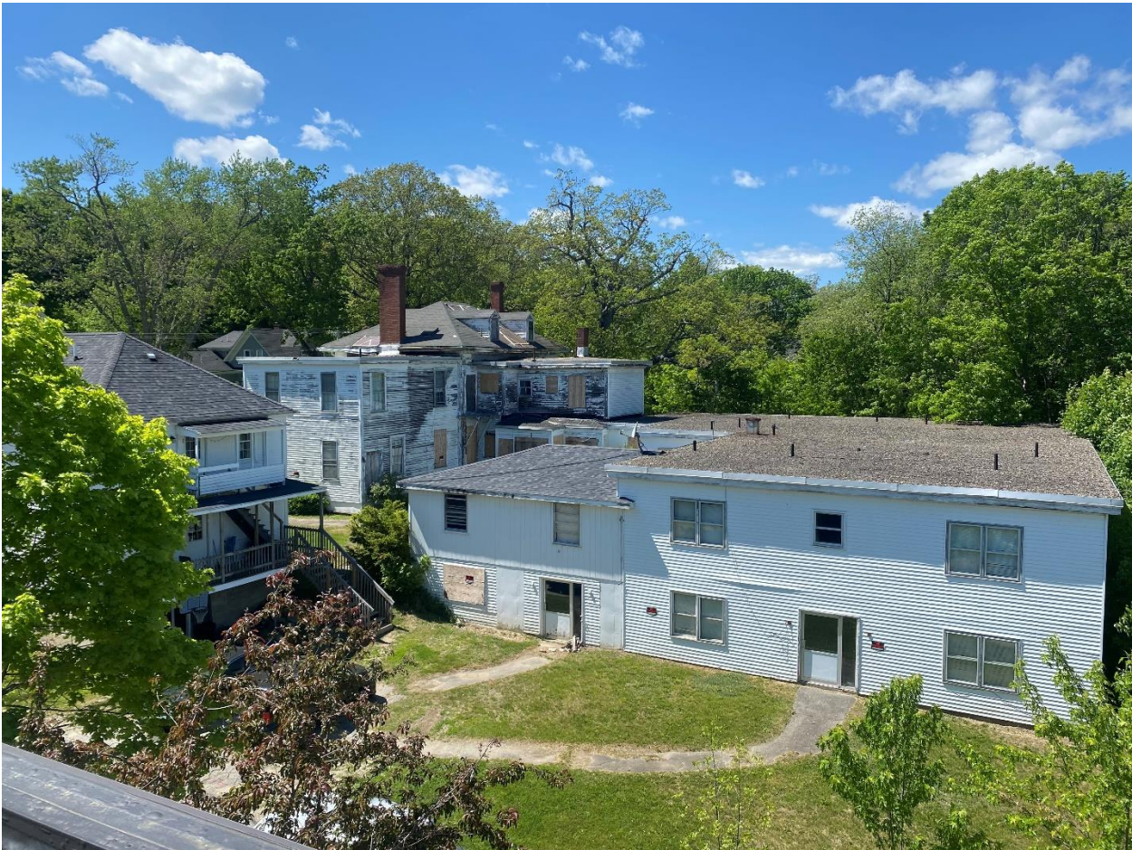
From the roof of Building 6 looking northwest at the abandoned Merrill Manor
