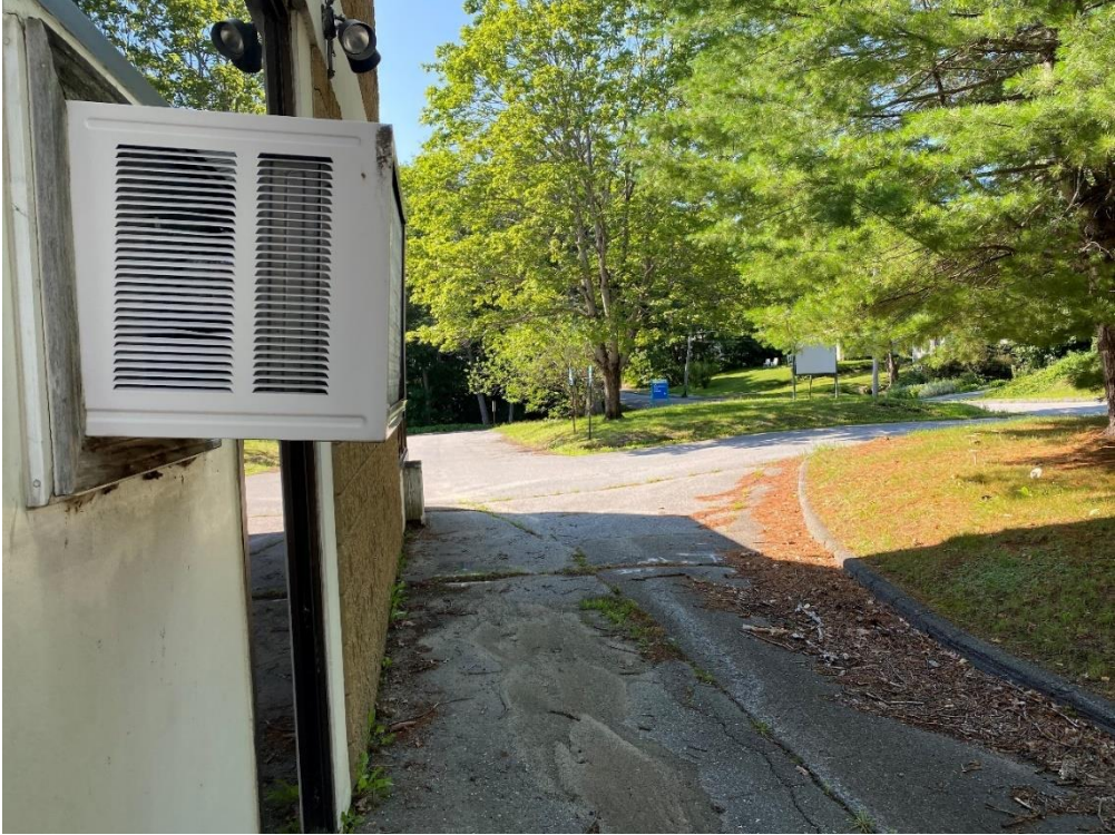
By the west facade of Building 6 looking south towards Dresden Ave.
