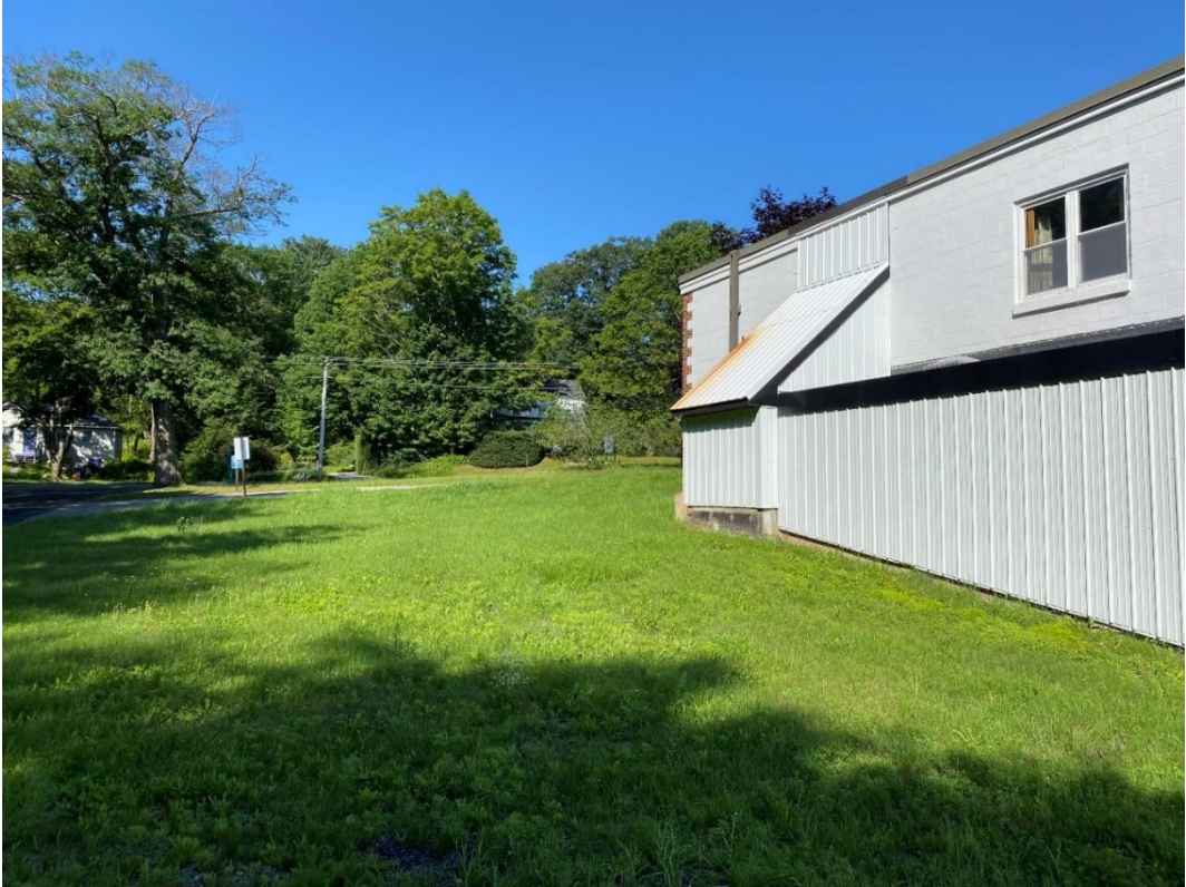
From the south of Building 5 looking north towards Dresden Ave.
