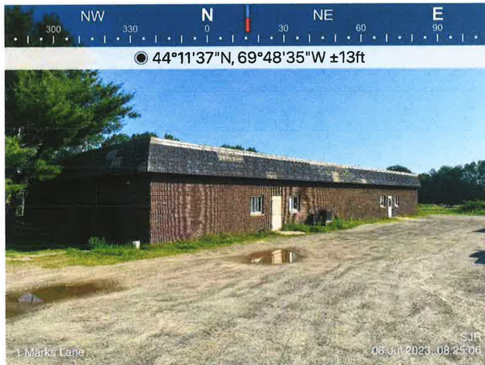
Existing site improvements include a commercial building and gravel parking lot
