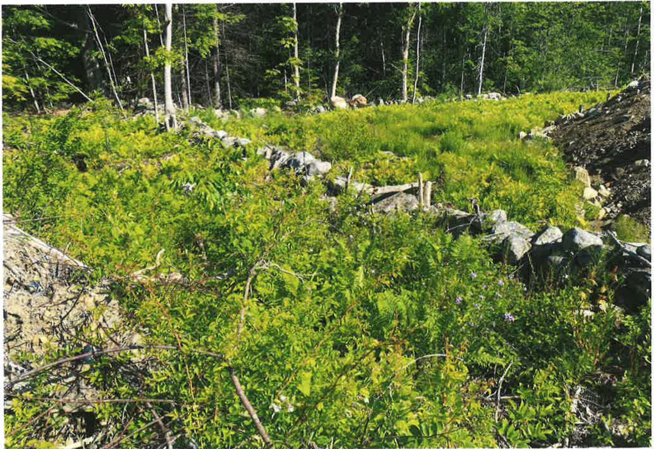
rock wall along rear of site
