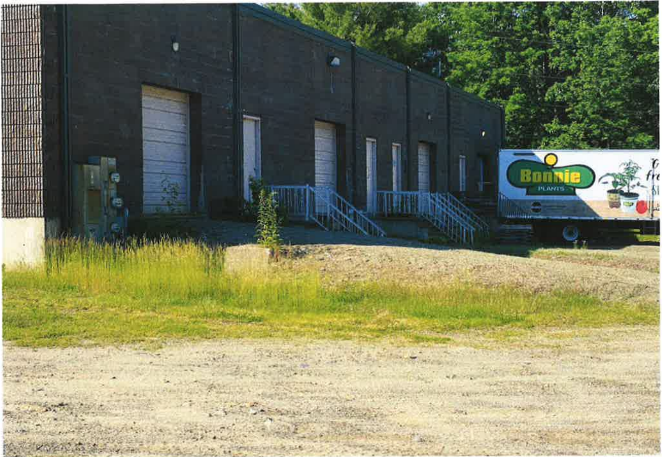
rear of building showing 3 loading areas and a drive up the ramp door. Each door has a mandoor.
