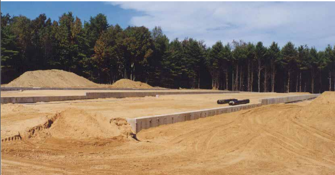
① FROST WALL DETAIL, NOTCHED
