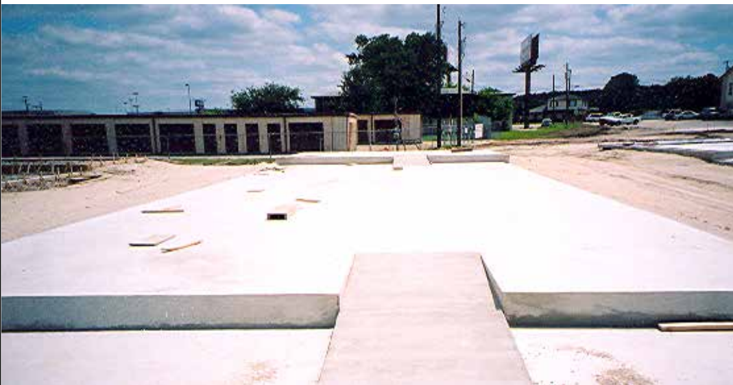
This ramp is centered in the step.
