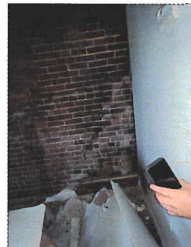
PHOTO 3 MAJOR STRESS CRACKS PENETRATED ALL THREE LAYERS OF BRICK NOTE UNSUPPORTED OPENING BELOW CAUSING FALLING BRICKS
