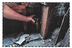
PHOTO 1 FALSE FRONT AT WATER STREET NOTE VISIBLE GAP TO THE EXTERIOR
