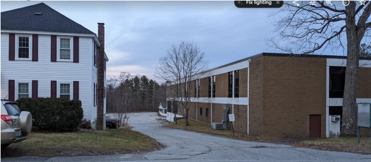
Existing north and west facades as viewed from Dresden Avenue:
