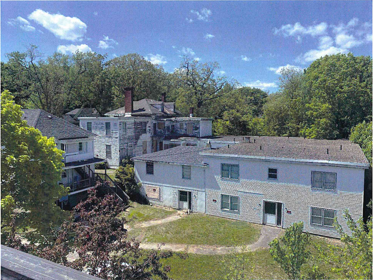
From the roof of Building 6 looking northwest at the abandoned Merrill Manor
