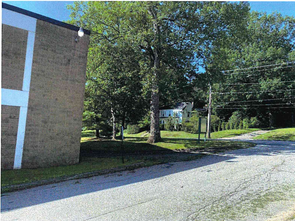
From the northwest corner of Building 6 looking southwest towards Dresden Ave.
