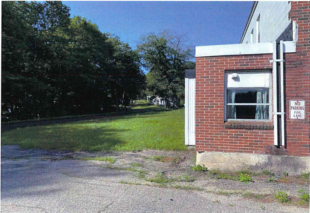
From the south of Building 5 looking north towards Dresden Ave.
