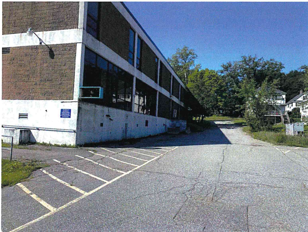
From the north of Building 6 looking west up the driveway. The abandoned Merrill Manor is to the right
