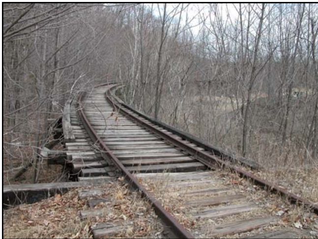
South end of the trestle, at the proposed trailhead area.
