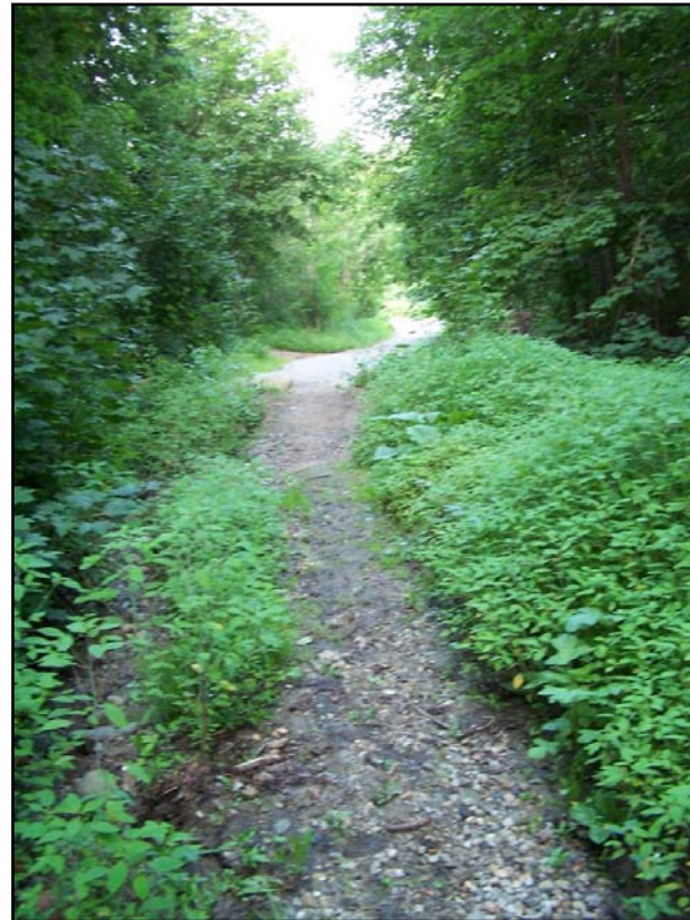
Harden "Street" is a City-owned ROW that connects Summer St. and Harrison Ave. The existing path is poorly constructed and in need of drainage improvements and erosion control.
